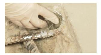
Concrete repairs can then be carried at any time after anode installation. There are no restrictions on the repair material to be used.
