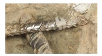
7. Apply a small amount of repair mortar to cap off the anode if the repair is not to be completed within 2 hours.
