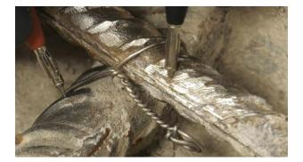
3. Drill 25mm (1") holes of the required depth at the edge of the patch repair (see table) making sure to avoid contact with the steel. Remove excess dust.
