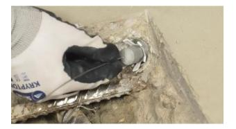
6. Connect the PatchGuard<sup>™</sup> by wrapping the anode tying wire (minimum 2 times) around the pre-cleaned steel bar and carefully tightening using pliers. This connection is essential for performance of the anodes.
